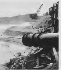
THE BEGINNING of a new dike, still a small ridge of sand, rises at the left over the inundated polder of Zierikzee. The mouth of a pipeline, which pumps sand to fill the area between the old and the new dykes, rests on a crumpled segment of an old dike.
